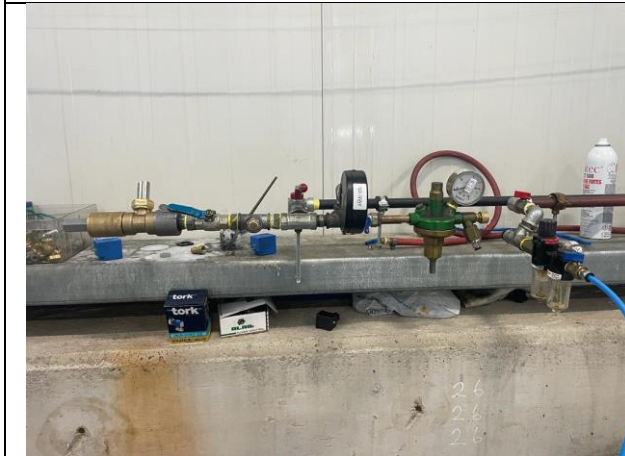
Pic.3 - Pressure Test Set Up
