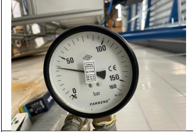
Pic.5 - Pressure Test
